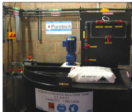
A view of the sodium hydroxide dissolution and storage tank.
